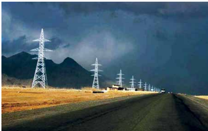
Transmission-line towers constructed by USAID between Arghandi and Ghazni. (USAID photo)
